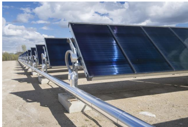
Σχήμα 3.2: Flat Plate Collectors for Solar Heat
